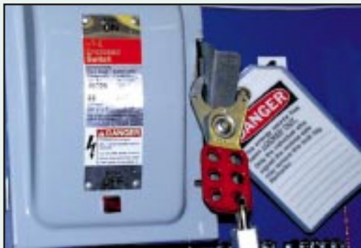
Always lock out and tag out circuits.
